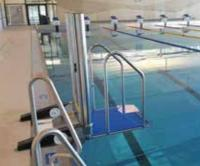
Hydraulic drive connected to water supply
